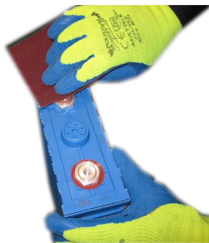
Picture 3.2.4.2: sanding the battery pole
